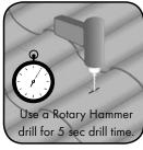
Step 10: Using a 1/2" carbide drill bit and ROTARY HAMMER DRILL in hammer mode, drill through the tile. See online video at www.prosolar.com for details.
